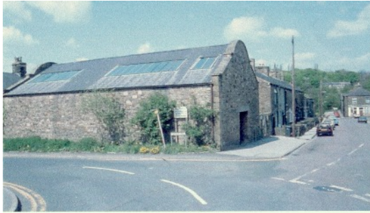
Fig 3 Newtown substation 331923. SJ 997850. opened in 1930 (Corner of Grove Road and Wirksmoor Road)
